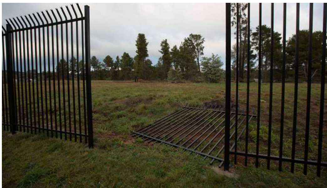
Fig.9 - Canberra Brickworks 23 June 2014 – new make safe fence not so secure....
