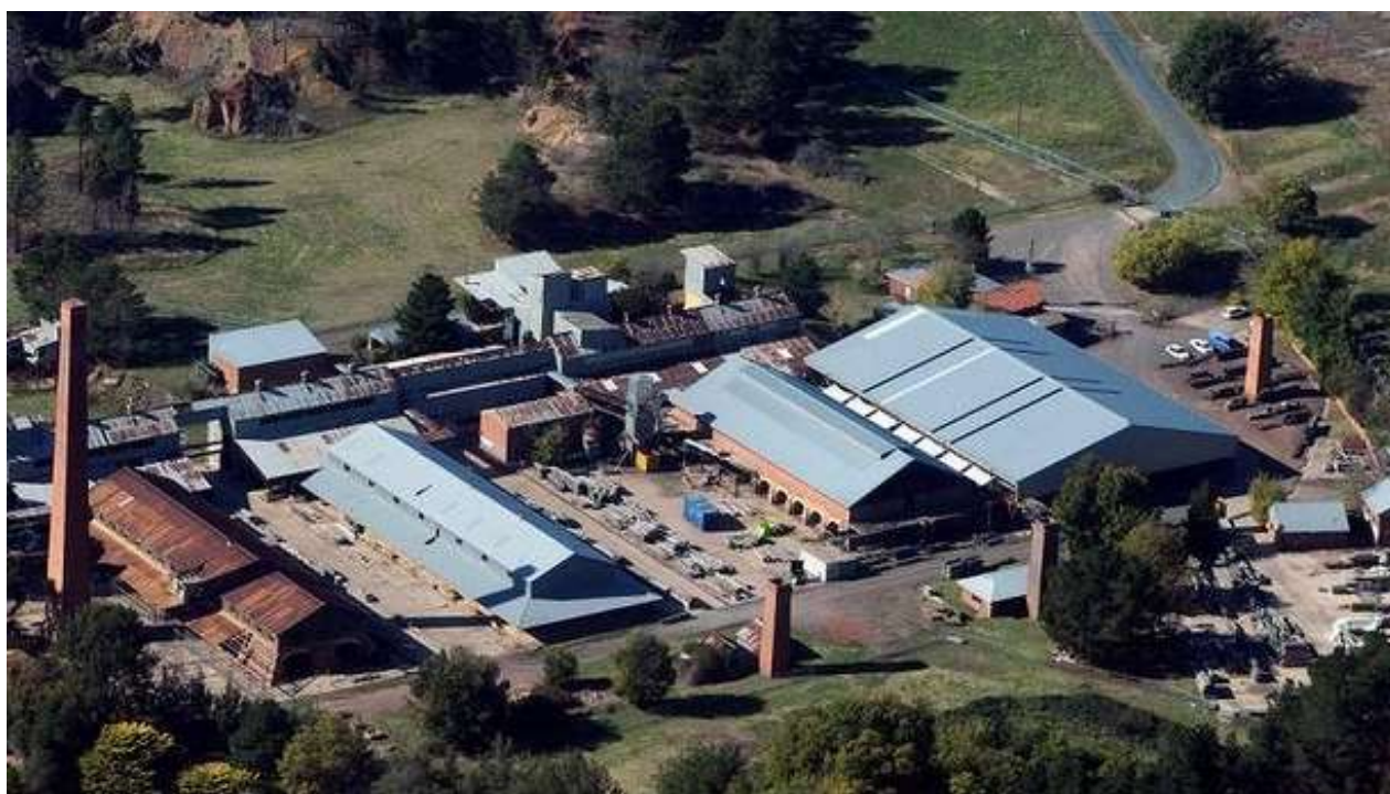
Fig.8 - Canberra Brickworks heritage buildings
