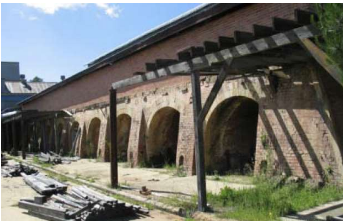
Fig. 10 - Condition of Canberra Brickworks buildings 2010
